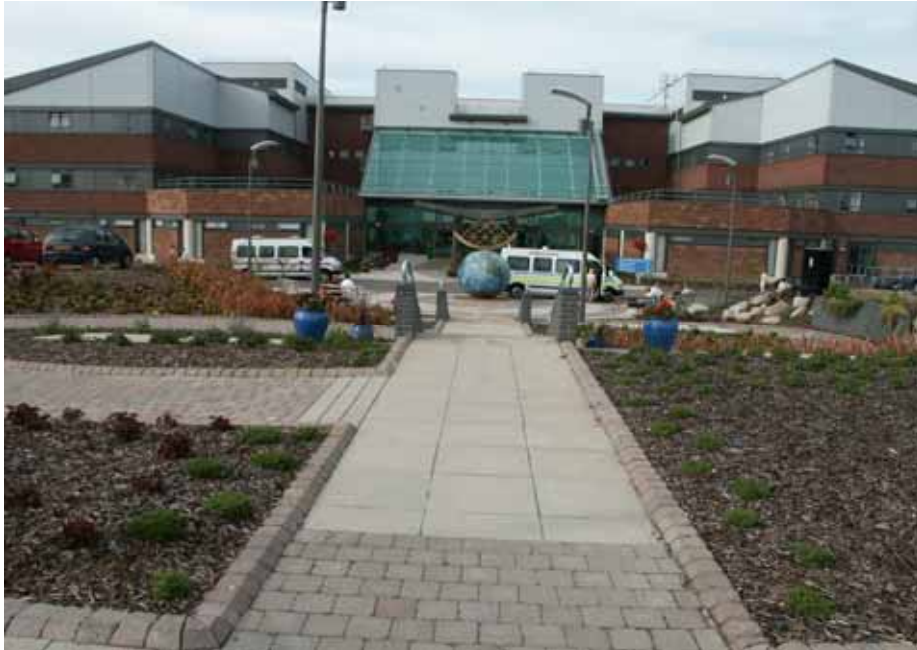
Fig 6.1: The new front entrance of the JCUH
