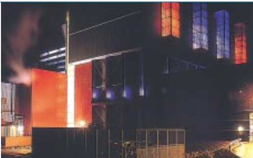
Martin Richman Energy from Waste Centre, Tyseley
