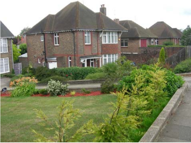
Detached 1930's houses in the Upper Drive
