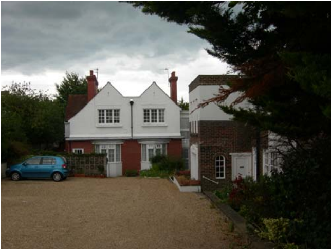
1930's house converted into flats opposite new development
