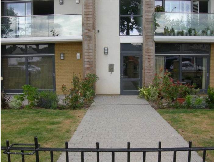
Front entrance to new development
