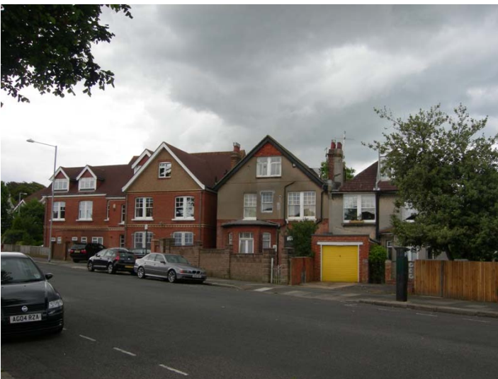
1930's housing in the Upper Drive
