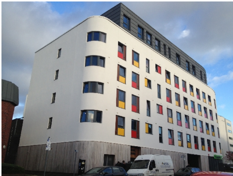
Above: Chesil House showing the external, ground floor, timber clad façade with its curved corner.
