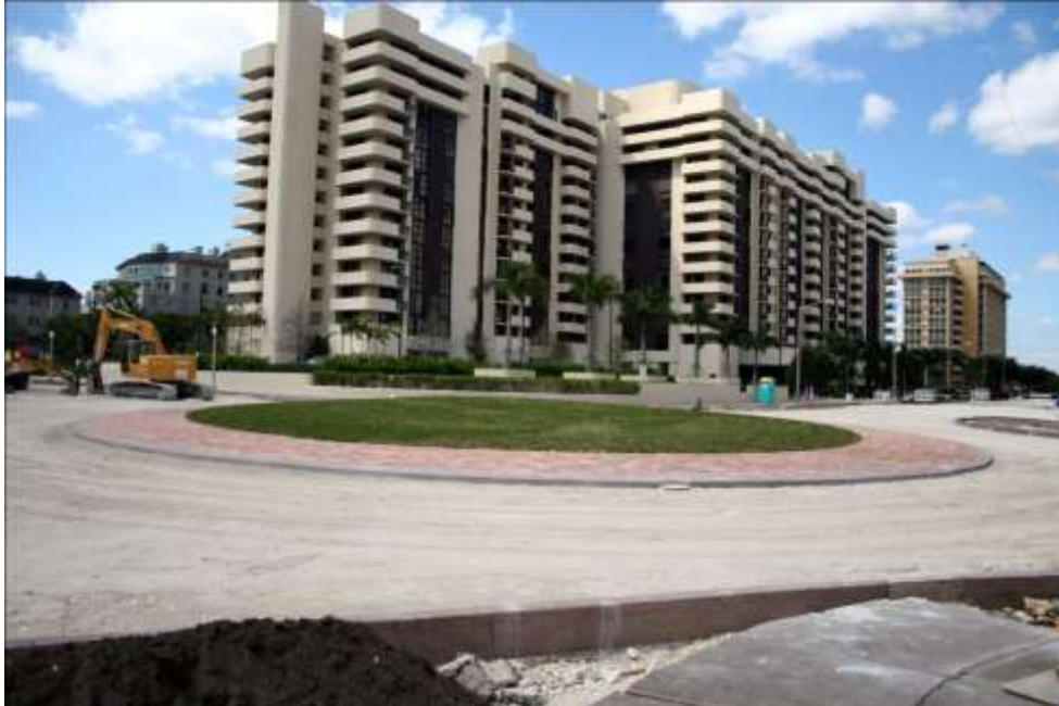
Intersection of Biltmore Way and Segovia Street. Pavers may be removed or changed, provided 5' from the back of curb is a structural material surface suitable to withstand vehicle loads.
