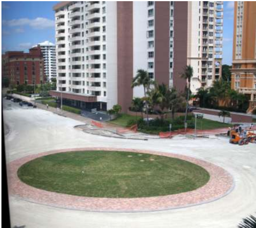
Intersection of Biltmore Way and Segovia Street. Pavers may be removed or changed, provided 5' from the back of curb is a structural material surface suitable to withstand vehicle loads.
