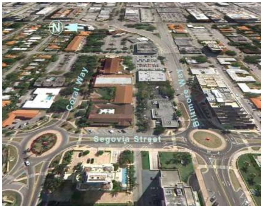
View looking to the East showing both circles. Photo does not accurately show the height of surrounding buildings.
