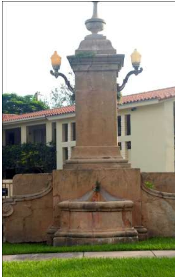
Existing Fountain Feature at Segovia Plaza.
