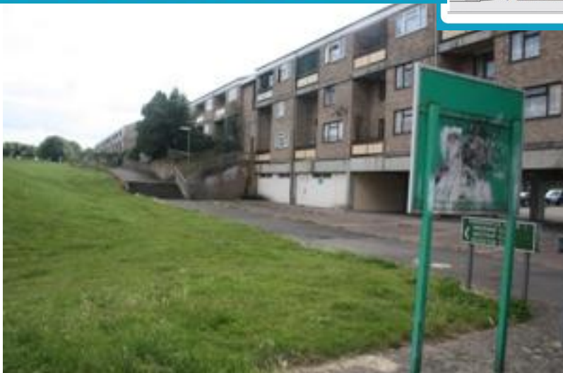
Figure 2 How the area looked before work began
