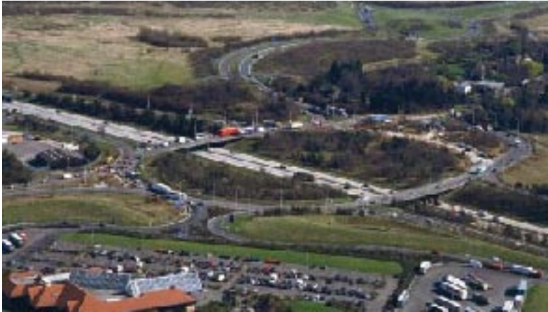
M11 motorway - junction 8. Image courtesy of BAA Aviation Picture Library.
